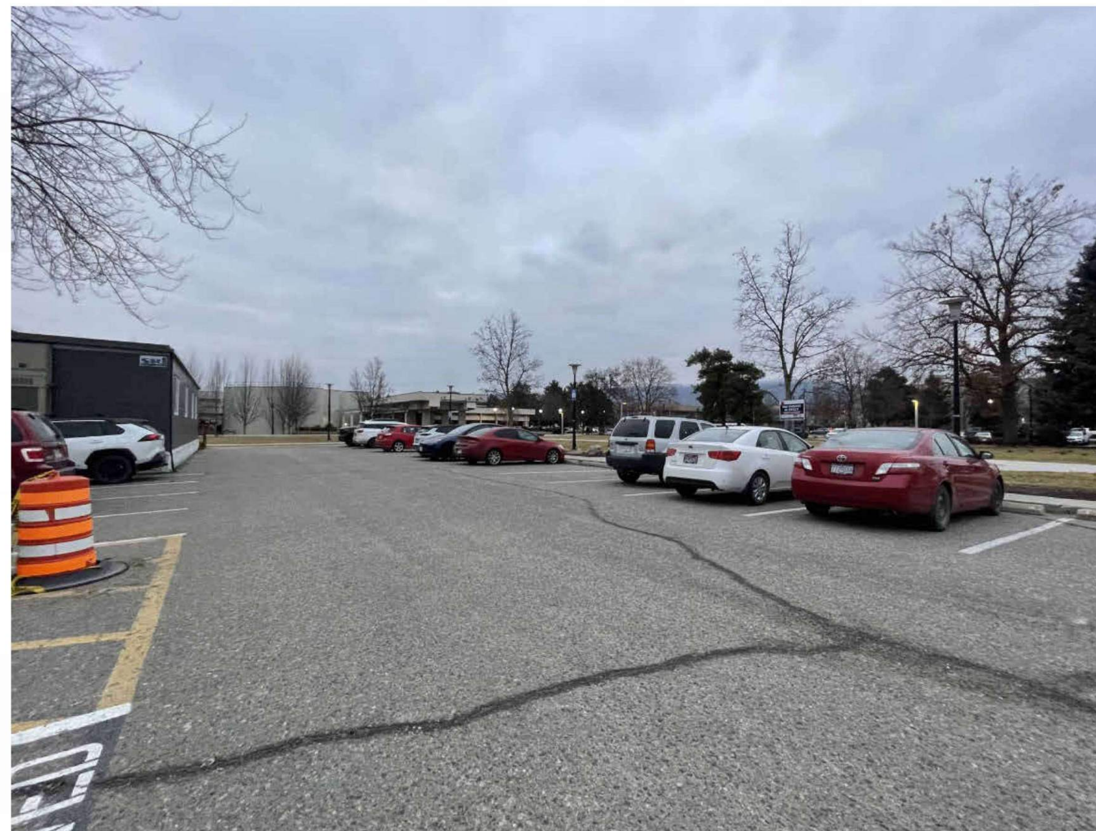
LOOKING SOUTH-EAST FROM EXISTING PARKING LOT
